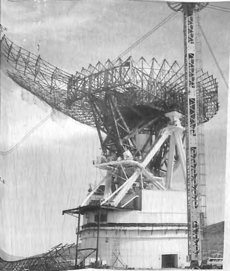
The radial rib back-up structure is installed for the 210-foot antenna.
