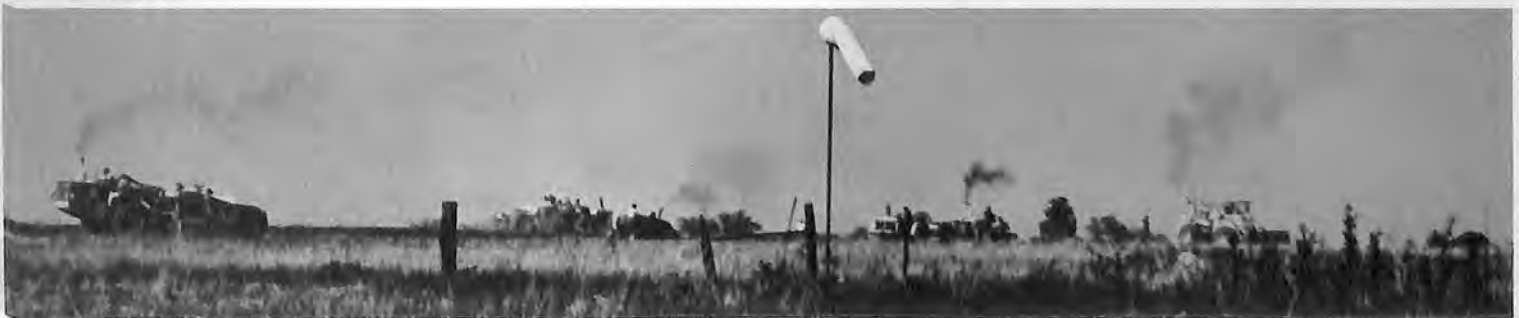
Windsock billows (below) as earth-moving equipment grades area.
