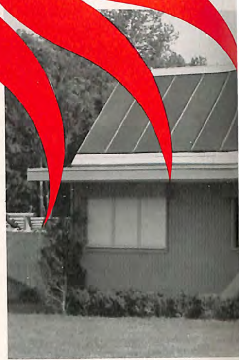
NASA's Tech House, located at Langley Research Center, Hampton, Virginia, incorporates a variety of advanced technology systems to cut home fuel consumption by two-thirds and water usage by half. Panels on roof are solar collectors, principal source of energy for home heating.
