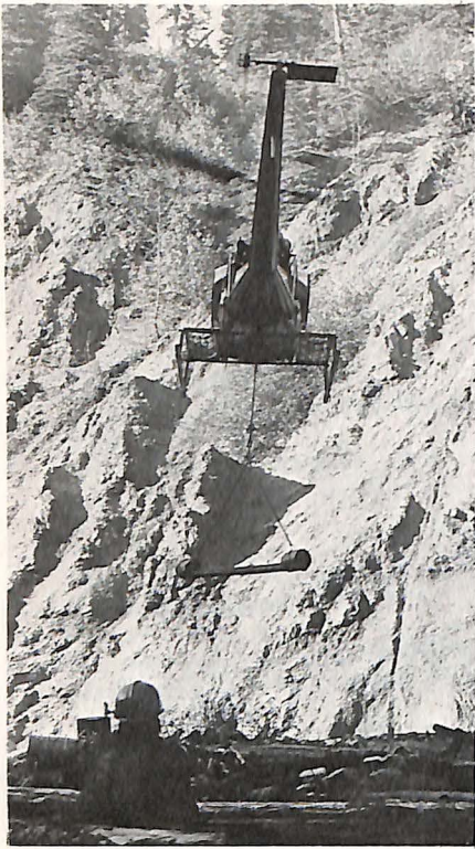
A Hiller 12E helicopter on the job high in the Rockies.
