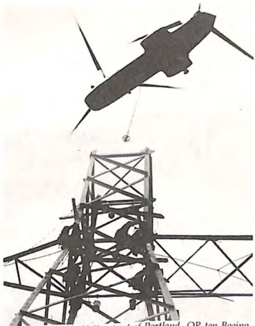
One of Columbia Helicopters' of Portland, OR ten Boeing Vertol 107-II helicopters erects a transmission tower in Indiana.
