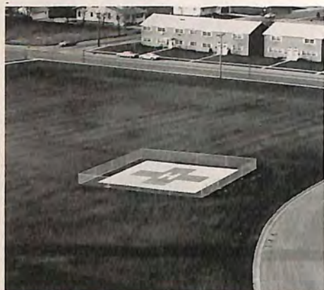
In a Joliet, Illinois residential, this 50' by 50' heliport is located near the emergency entrance at St. Joseph Hospital.
