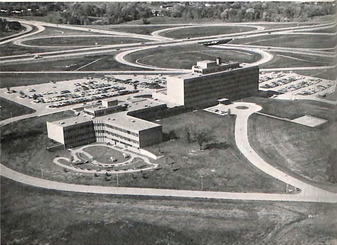
The Missouri Baptist Hospital heliport in St. Louis County, MO.
