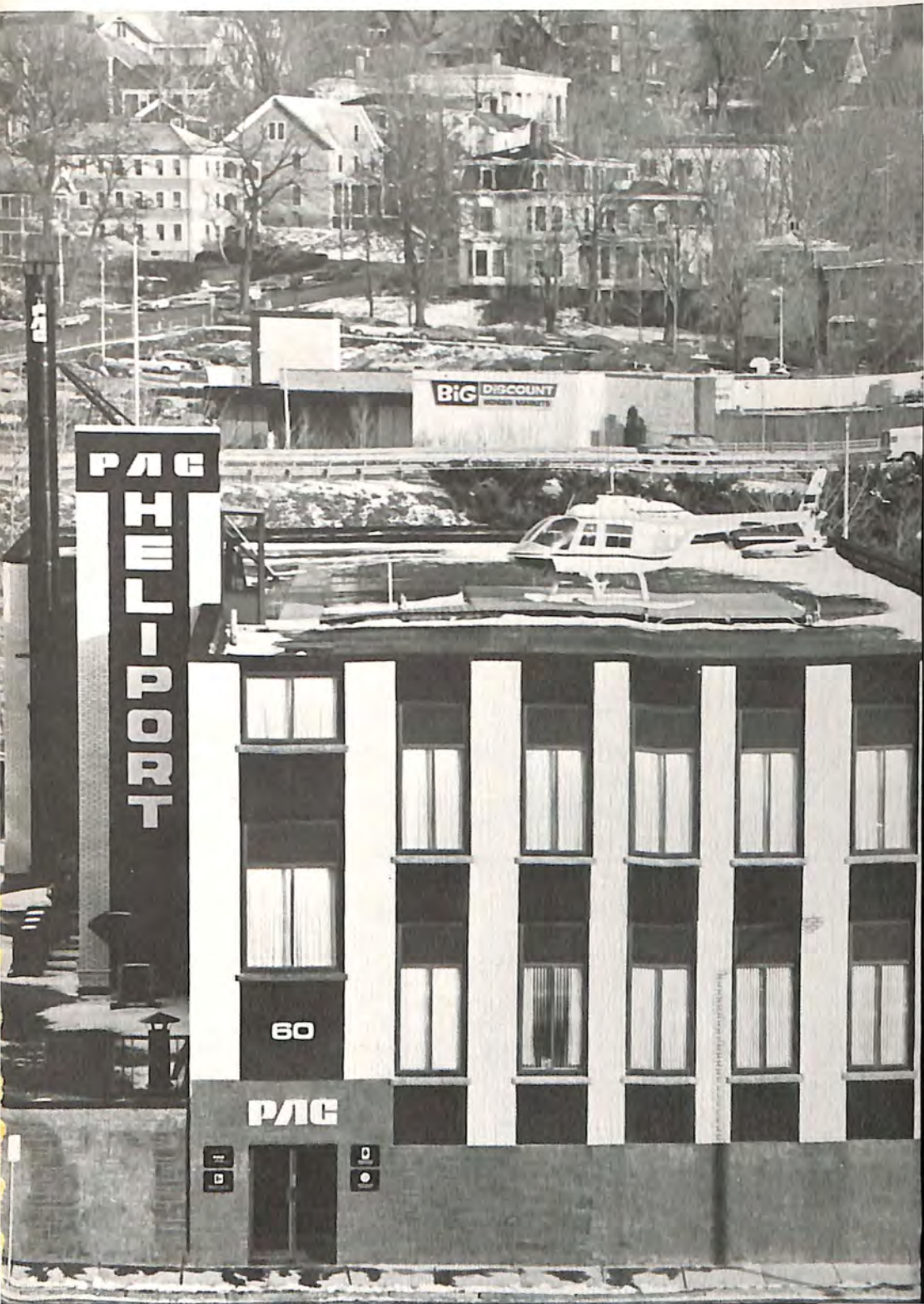
In Worcester, Massachusetts, one of the Parker Aviation Corp's Bell JetRangers lands on the company's rooftop heliport.
