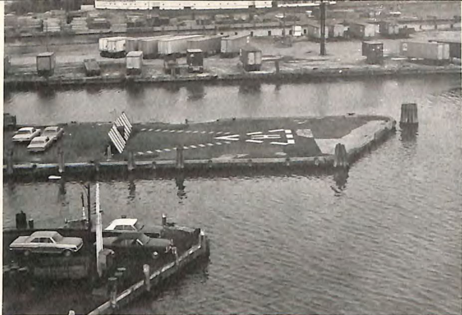
Pier 4, Baltimore, Maryland's downtown, public heliport.
