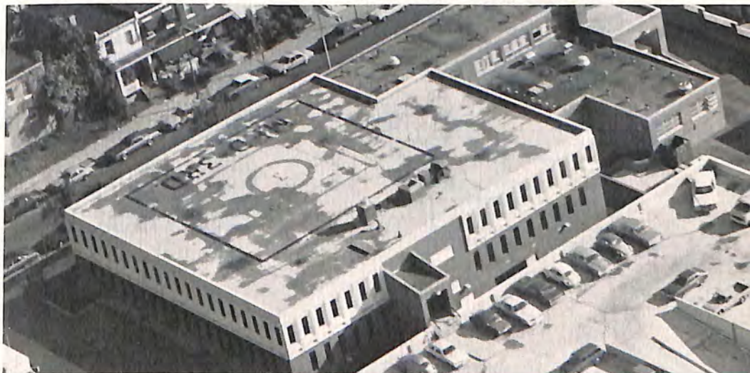
In Washington, D.C., one of the Metropolitan Police Department's three rooftop heliports.
