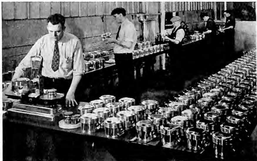
Final inspection of aluminum pistons for Wright Cyclone aircraft engines. EXACT WEIGHT Scales handle this particular operation in one of America's leading motor car plants.
