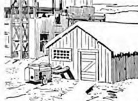
Supplying emergency heat to buildings
