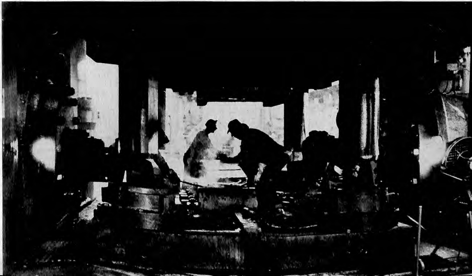
Forging structural aircraft components on the Wyman-Gordon 35,000-ton press.
