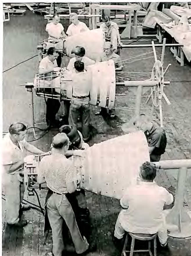
Thrust chambers of XLR-115 engines.
