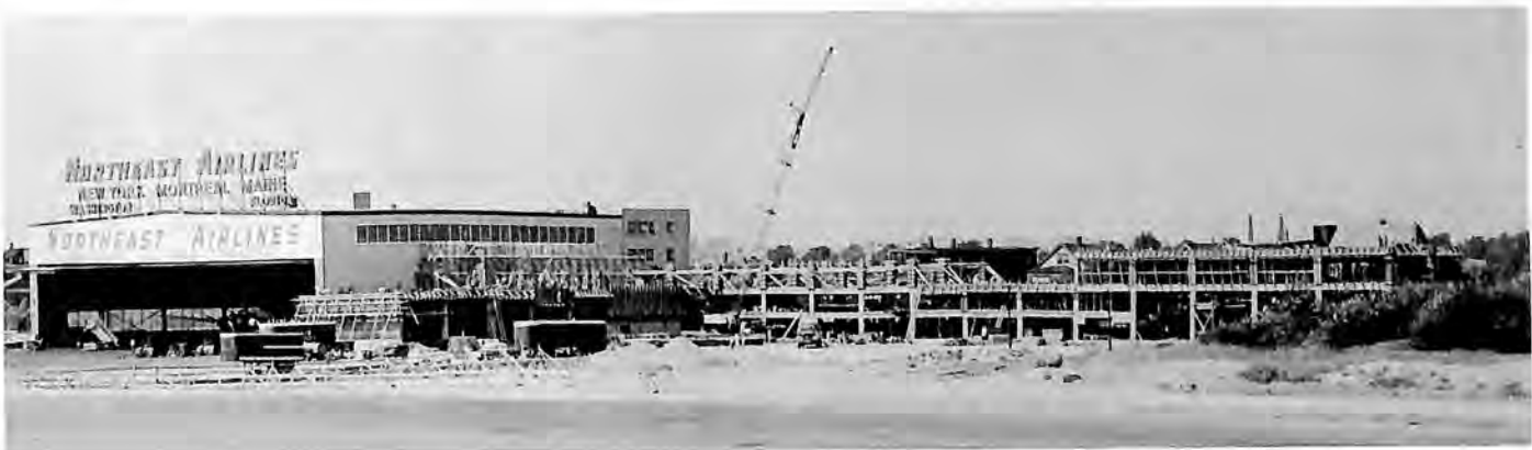
New facilities for Northeast were being constructed at Logan Airport.
