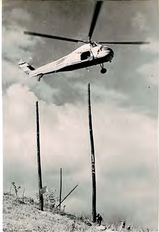
Sikorsky S-58 sets huge power line poles.
