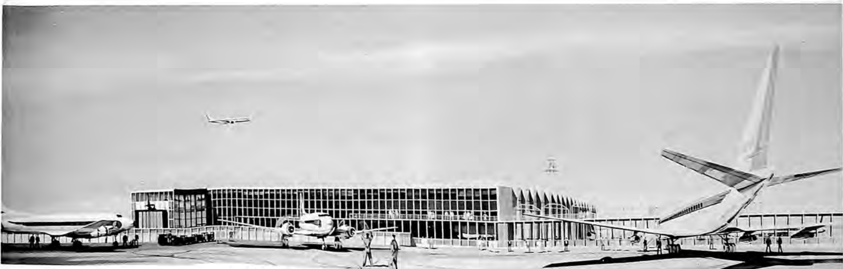
Eastern's new passenger terminal was under construction at Idlewild.
