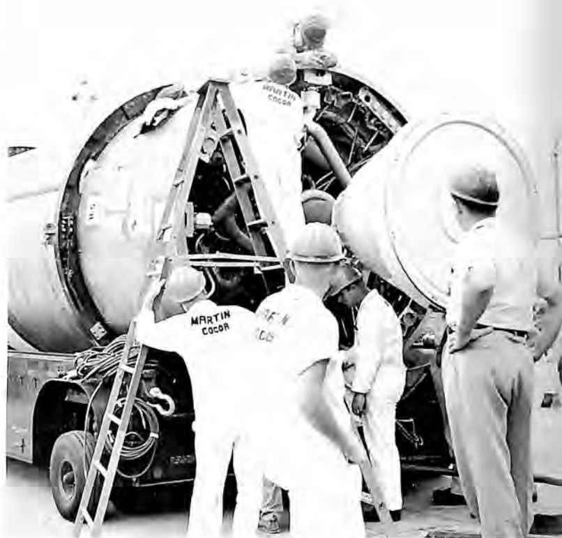
Technicians prepare second stage of Titan for erection on launch stand at Cape Canaveral.
