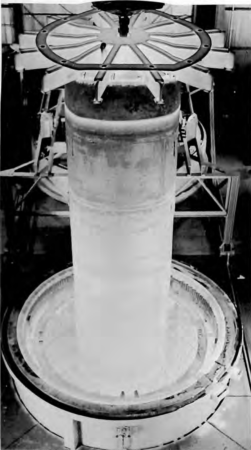
Rocket motor case emerges from Solar furnace.
