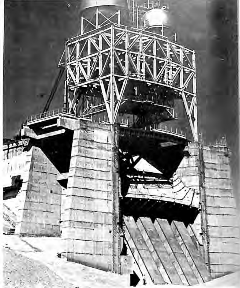
Completed in 1961 was world's largest rocket engine test stand, for test of Rocketdyne's 1,500,000 pound thrust F-1 engine.
