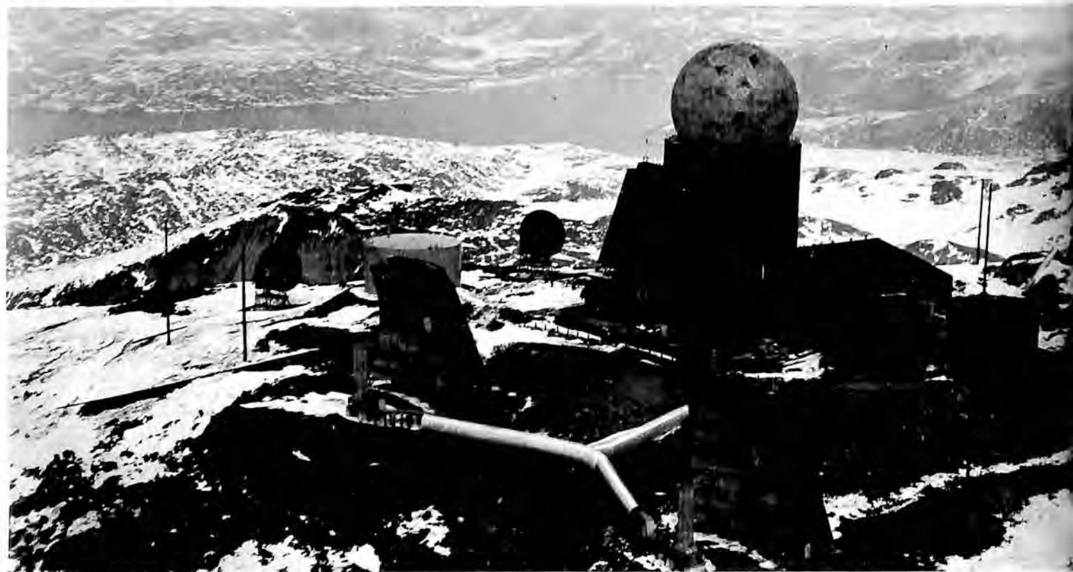
A DEW Line station, "DYE-1," located on the western shore of Greenland. Western Electric was prime contractor for engineering, installation and testing of the DEW East project's electronics and communications services.
