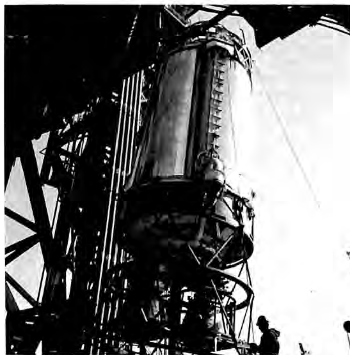
Centaur stage is readied for mating with Atlas booster.
