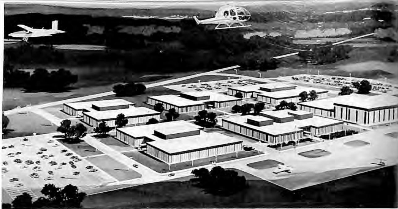
Construction started on Fairchild Hiller's Sherman Fairchild Technology Center, scheduled for completion in late 1966.
