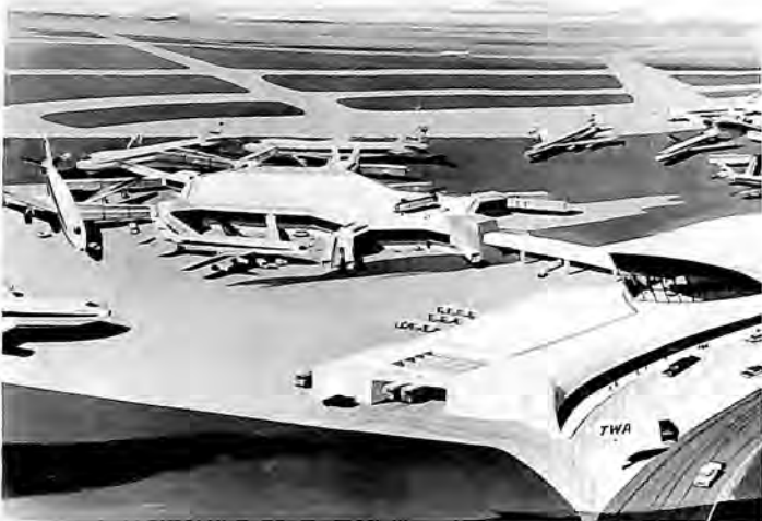
Work started on TWA's Flight Wing One, the $19,800,000 "Terminal of Tomorrow," to be opened in 1969 for use by Boeing 747s and, later, SSTs.
