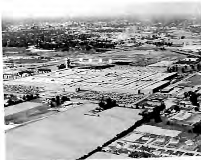
Allison added nearly 250,000 square feet of manufacturing area to its principal gas turbine engine production facility.
