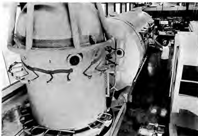
The Cachalot-850 prolonged submergence or saturation diving system is outfitted at Westinghouse Underseas Division's Ocean Research and Engineering Center for dives to depths of 1,000 feet.
