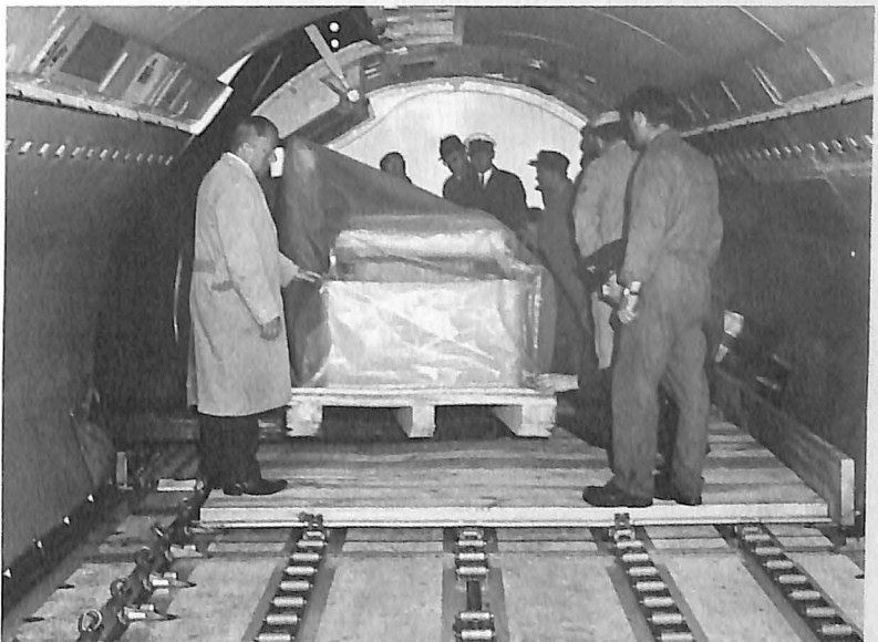
Under plastic wraps, profile borer unit mounted on skid is carefully hoisted through front cargo door of Lufthansa jet freighter during night loading at Stuttgart.
