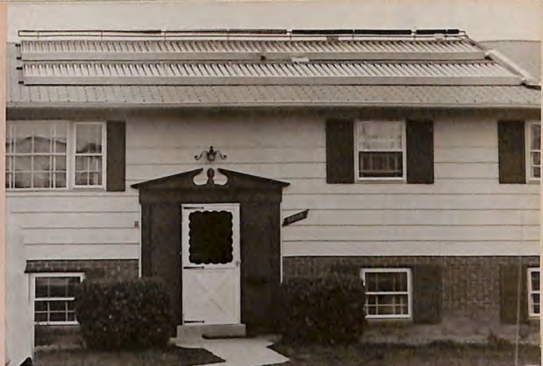
At left, Grumman solar collectors enhance home design while capturing sun energy for home heating. Photo at right shows an experimental installation of a new General Electric solar array which uses vacuum tubes rather than the customary glass plates to trap solar radiation.
