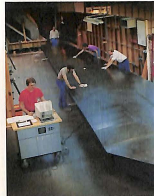
Rockwell-Tulsa fabricated a 50-foot layup tool as part of the Air Force/Rockwell Large Aircraft Composite Wing Structures (Mantech) program.
