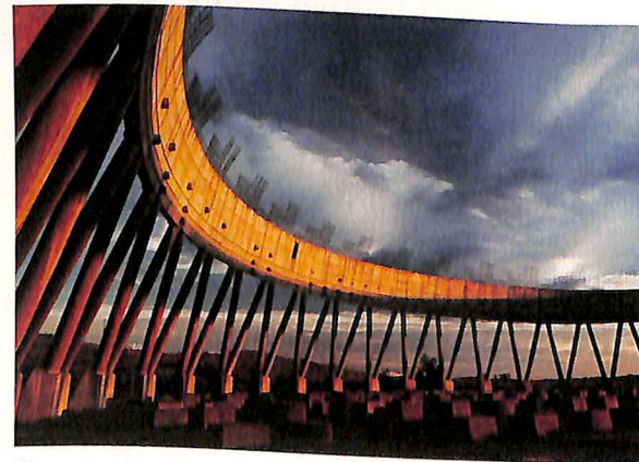
Shown here is a cooling tower foundation that is being converted to storage facility for NASA's Advanced Solid Rocket Motor (ASRM) at Yellow Creek, Mississippi. Groundbreaking ceremonies were held in April for conversion of the never-completed nuclear facility to a production plant for the ASRM, being built by Aerojet under contract to Lockheed Missiles & Space Company.
