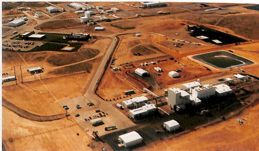
AMERICAN PACIFIC CORPORATION A pioneer in the use of ammonium perchlorate as a rocket fuel component, AMPAC built a new perchlorates production complex in southern Utah (shown). At the same site is a new plant for manufacture of sodium azide, the inflation chemical in automotive safety bags and fire suppression products.
