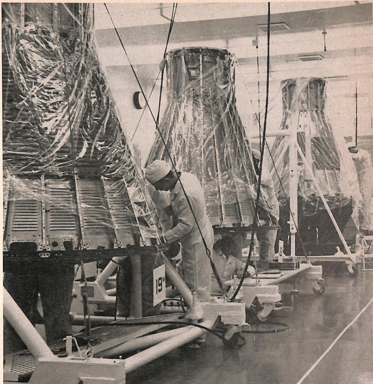
Mercury capsules are fabricated under superclean hospital-like conditions to insure against clogging of systems by foreign particles. Even the tiniest dust mote is a potential source of malfunction.
