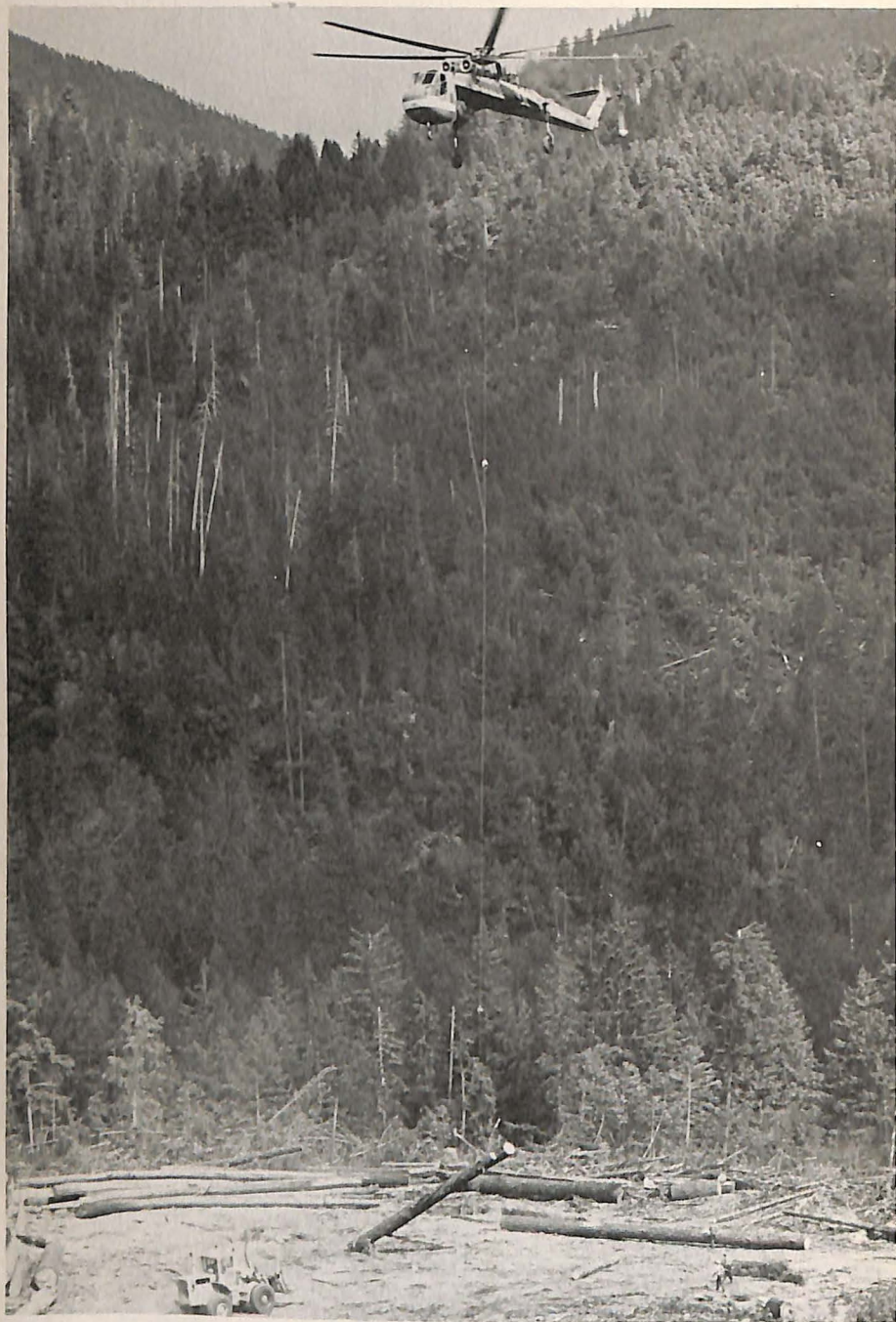
Erickson Air Crane Company of Marysville, Cal. -- first commercial operator of the Sikorsky S-64E -- SKYCRANE -- shown here loading felled lumber in Oregon's Siskiyou National Forest.
