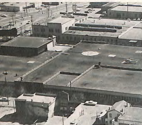
The Coco Cola building's rooftop heliport in downtown Dayton, Ohio provides hangar space, fuel and maintenance. It was the first rooftop facility to have these services.
