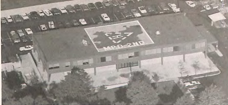
2nd DISTRICT-3320 IDAHO AVENUE, N.W.
