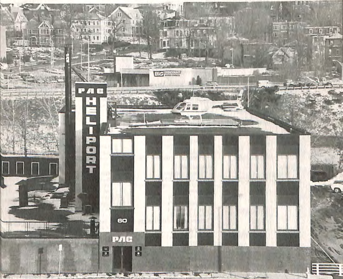
In downtown Worcester, MA, the Parker Aviation Corporation's rooftop heliport.
