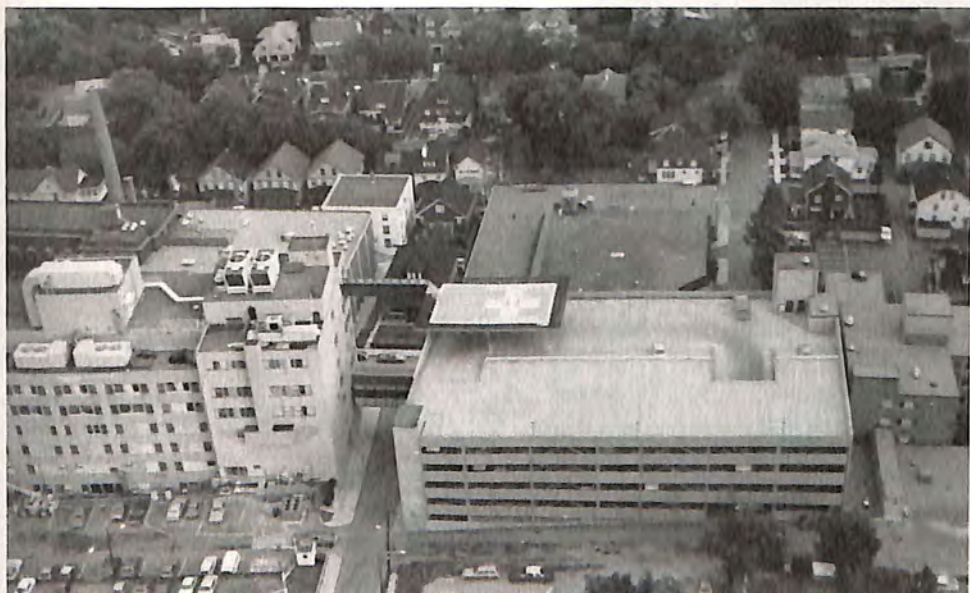
The Conemaugh Valley Memorial Hospital Rooftop Helistop in Johnstown, Pennsylvania. (Heliport Systems, Inc.)
