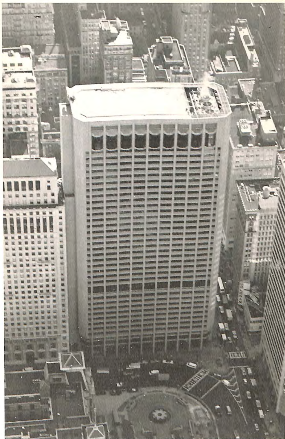
In downtown Philadelphia, Pennsylvania, the Girard National Bank rooftop helistop. (Heliport Systems, Inc.)
