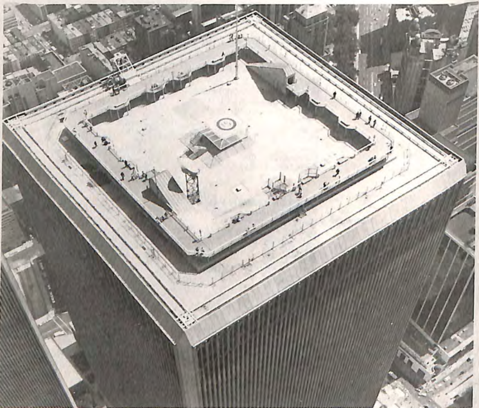
In New York City, the World Trade Center's emergency evacuation rooftop helistop.
