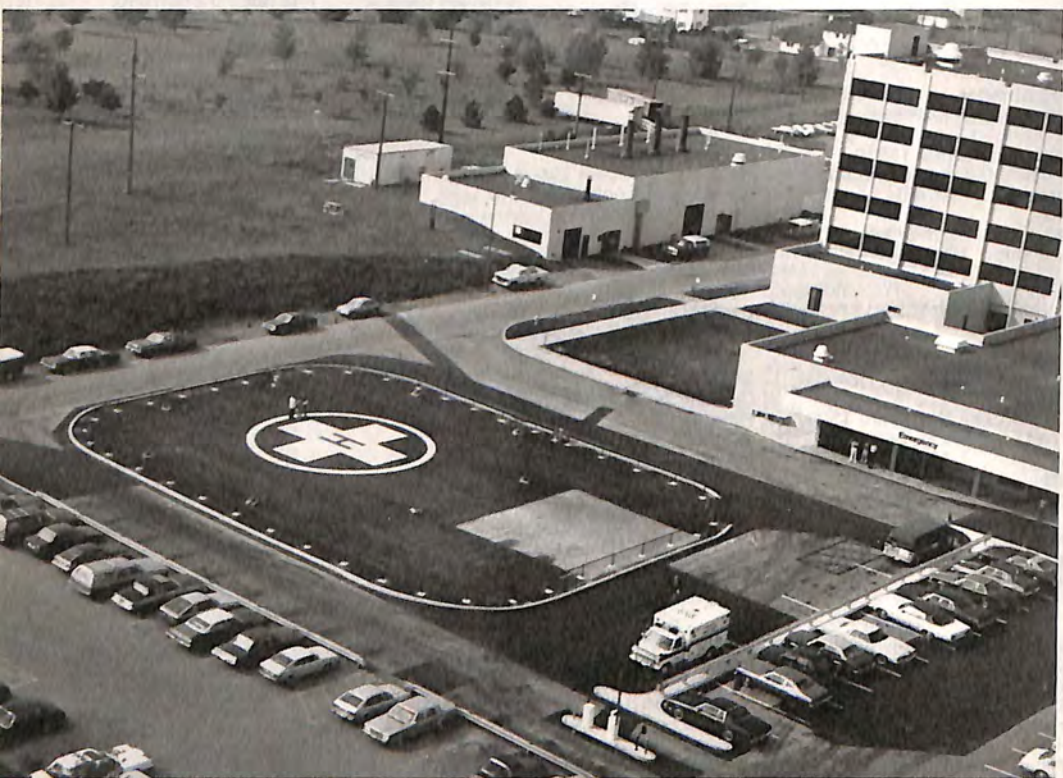
In Pennsylvania, the new Trauma Center Helistop at the Allentown and Sacred Heart Hospital Center.
