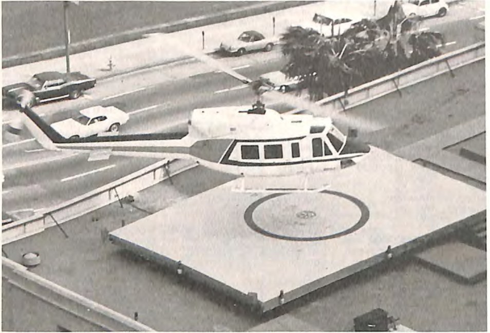
A Bell 212 hovers over the Los Angeles, California City Hall rooftop heliport.
