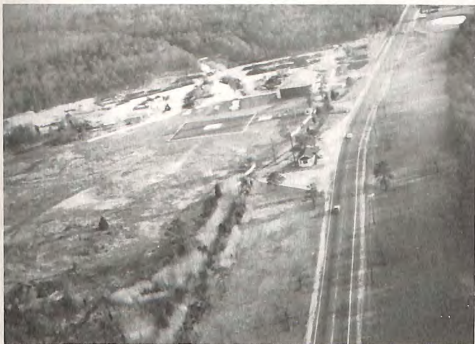
The new public use Germania Heliport in Pomona, New Jersey, provides full service (fuel, maintenance, hangar parking) for transient helicopters operating in and out of Atlantic City.
