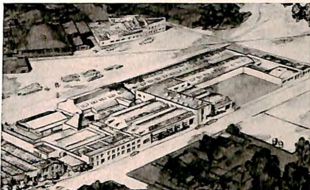
LOS ANGELES OFFICES AND FACTORY OF CANNON ELECTRIC
