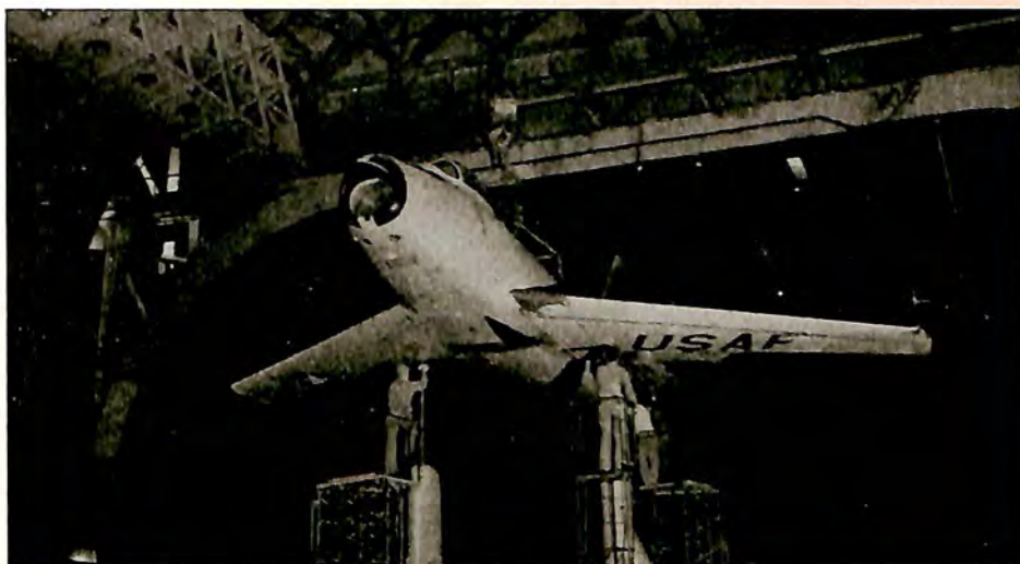
North American F-86 being readied for wind tunnel tests
