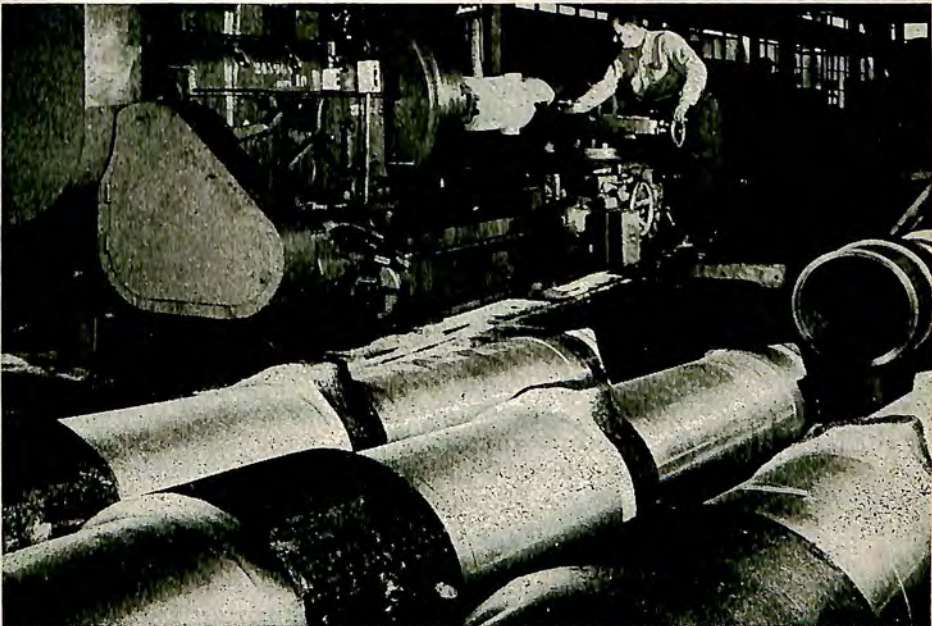
Main leg columns for B-36 in Cleveland Pneumatic Tool Co.
