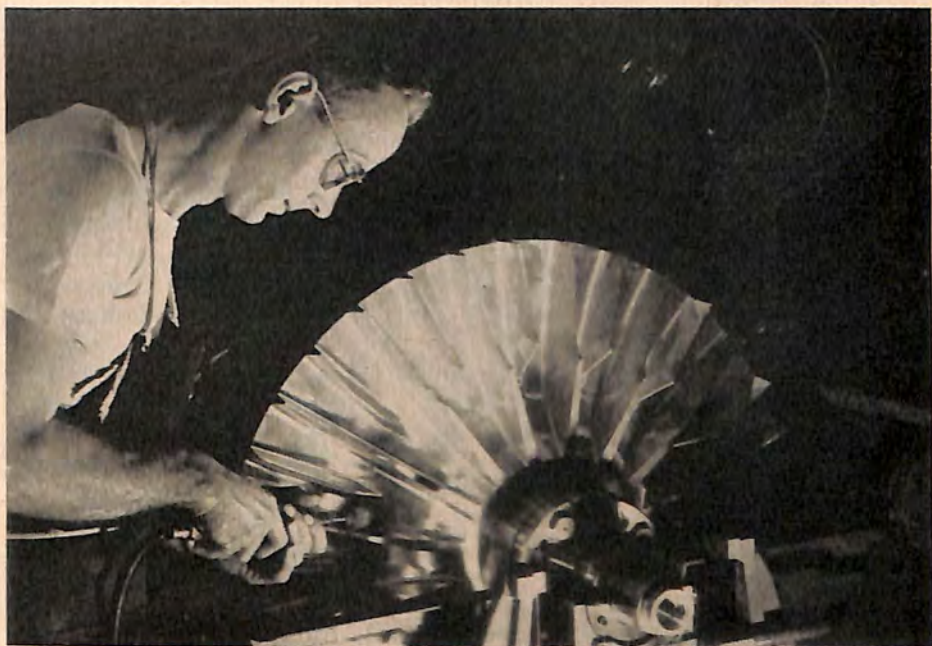
Allison employee removes burrs from impeller of J33 turbojet engine compressor
