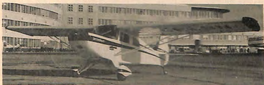
New Taylorcraft model features fibreglas reinforced plastic exterior
