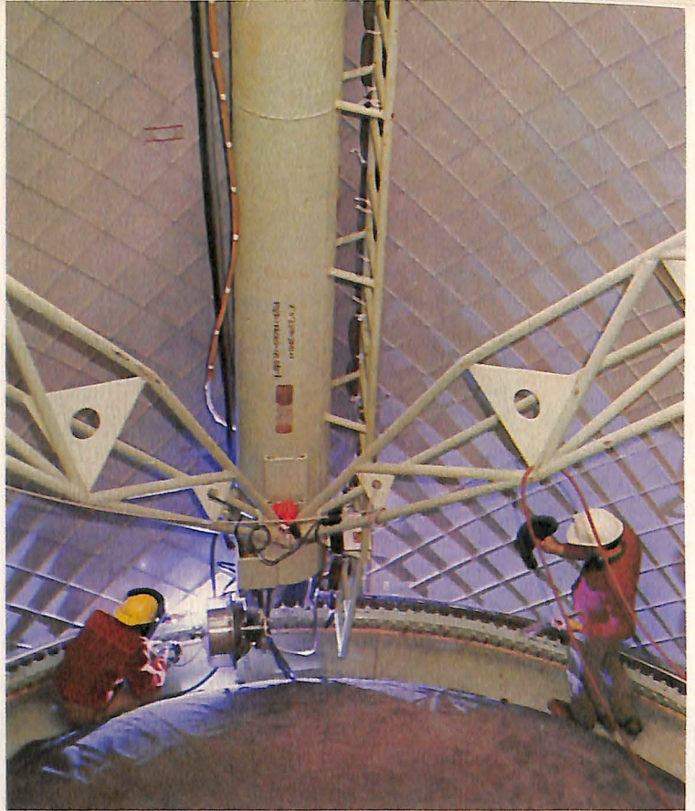
Douglas Aircraft Company technicians weld a section of a Saturn booster stage.
