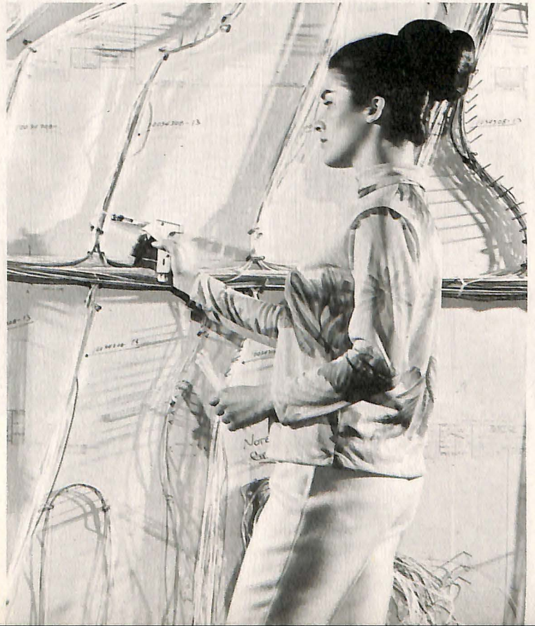
A Bendix Corporation technician uses a special gun to bond plastic loops around electrical circuits.
