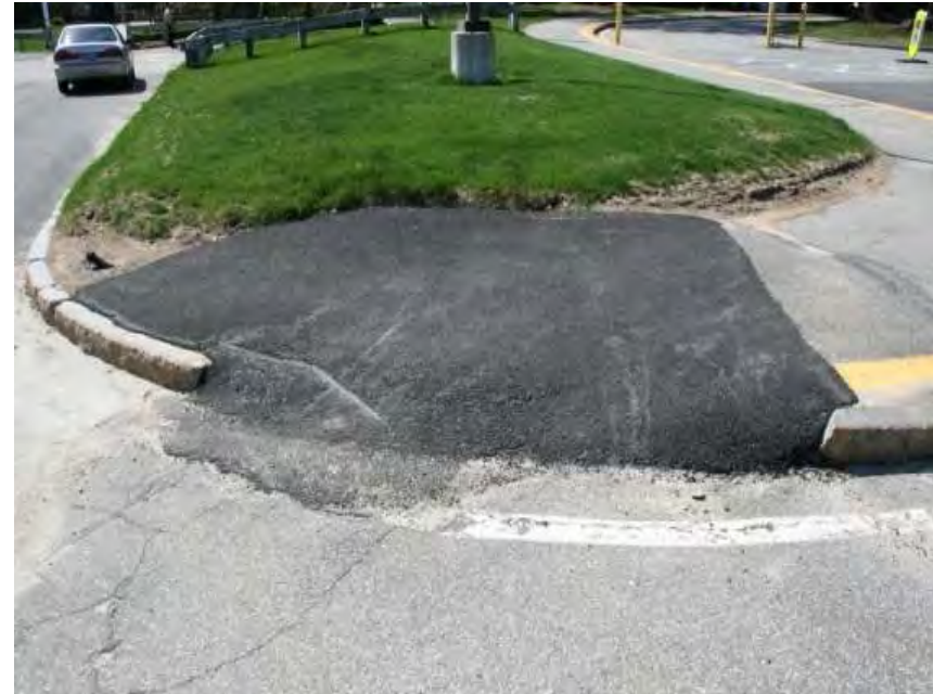
Placement of Curb Cuts
