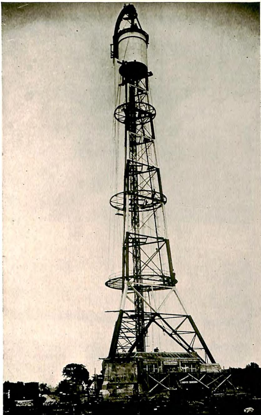
Two hundred and ten foot airship mooring mast designed and constructed by Aircraft Development Corporation at Ford Airport, Detroit, Mich. Similar mast being constructed by Aircraft Development Corp. for U. S. Army at Scott Field, Belleville, Ill.
