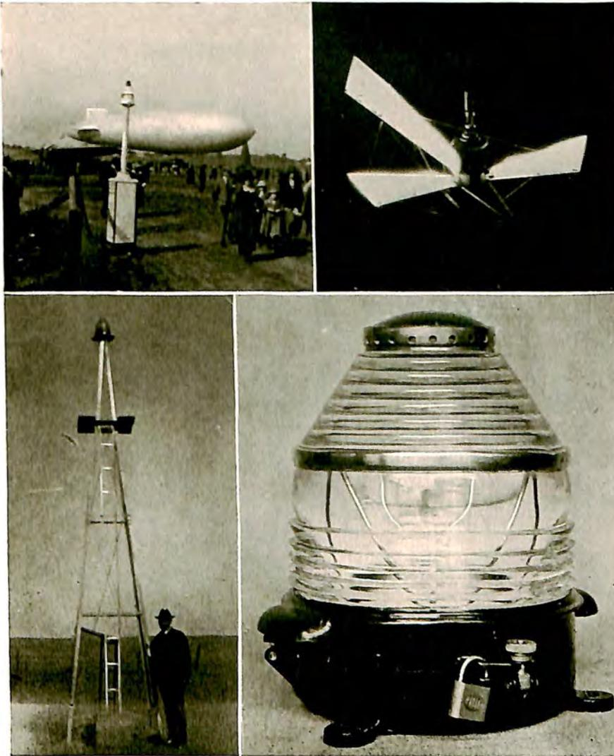
(Top Left) American Gas Accumulator Route Beacon used by Army Air Service and Air Mail. (Top Right) AGA illuminated wind indicator. (Bottom Left) Interflash Signal Corporation's Aerial Beacon used by Army Air Service and Air Mail. (Bottom Right) Close-up of Interflash Beacon, visible 360 degrees and 180 degrees through the vertical; operates one year without attention.
