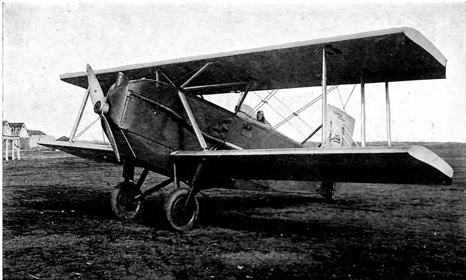
Curtiss Aeroplane & Motor Company's *Carrier Pigeon*. This new type cargo airplane carries 1,000 lbs. of mail or express, has radius of 500 miles and a top speed of 126 m.p.h.
