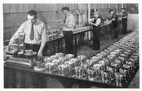
Final inspection of aluminum pistons for Wright cyclone aircraft engines. EXACT WEIGHT Scales handle this particular operation in one of America's leading motor car plants now devoted to complete war production.
