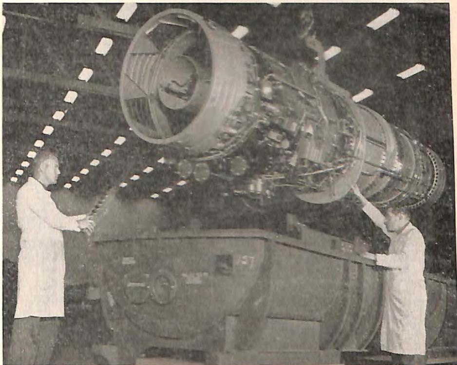
bustor liners and a four-stage turbine. It weighs 1610 pounds and is 145 inches in length, 27 inches in width. The AeroProducts propeller is of hollow steel construction and measures 13.5 feet in diameter.
