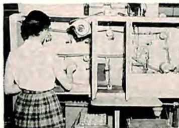
All sealed relays are thoroughly cleaned of dirt, solder flux and other contaminants by the ultrasonic cleaning process.
