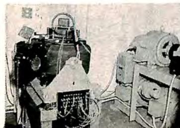
Servo controlled shaker and rotary power supply located in sound-proof room has frequency range of 0 to 2,000 C.P.S.
