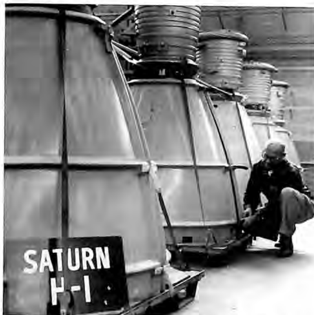
ROCKETDYNE Model H-1 Rocket Engine Thrust Chambers
