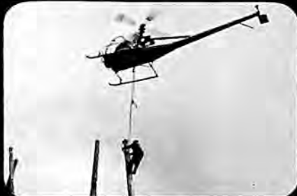
12 E, first light copter to erect entire powerline; 40' poles, el. 5,000 ft.
