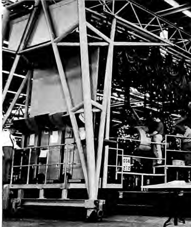
ELECTRICAL testing harness draping over an F-105D fuselage from bridge-like frame.
