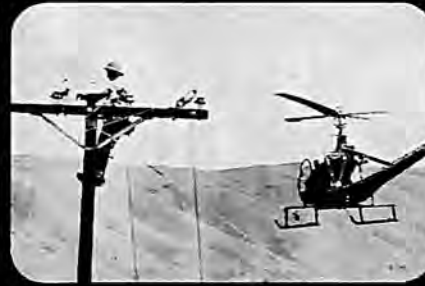
2½ mile powerline built in 6 hrs., 50 mins. with E's 305 hp at work.
