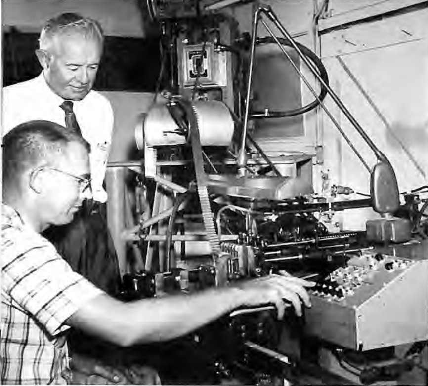
FRED H. ROHR, founder and chairman of the board, supervises operation of new stainless steel honeycomb core manufacturing machine.
