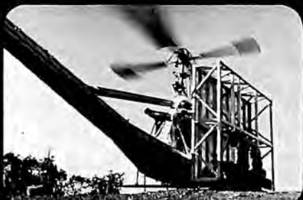
Microwave station on 4,000' ridge; all 8 tons material; 2 days flying.
