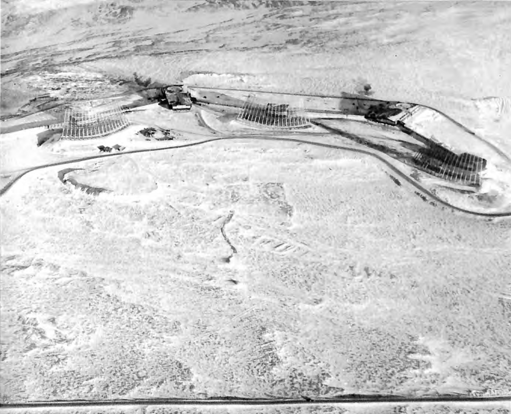
PANORAMIC VIEW of the first Ballistic Missile Early Warning System (BMEWS) site, Thule, Greenland.
